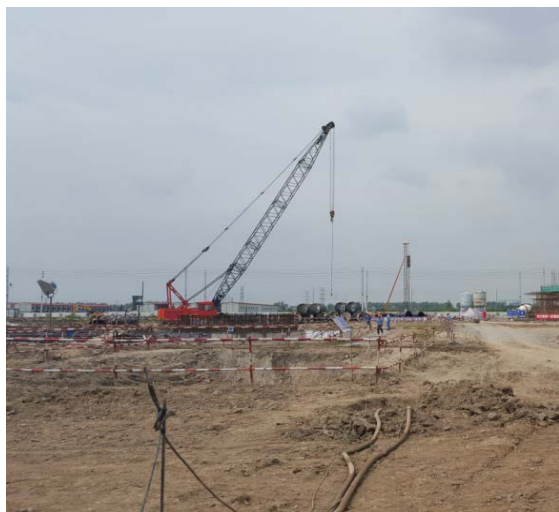
厂区土方开挖
